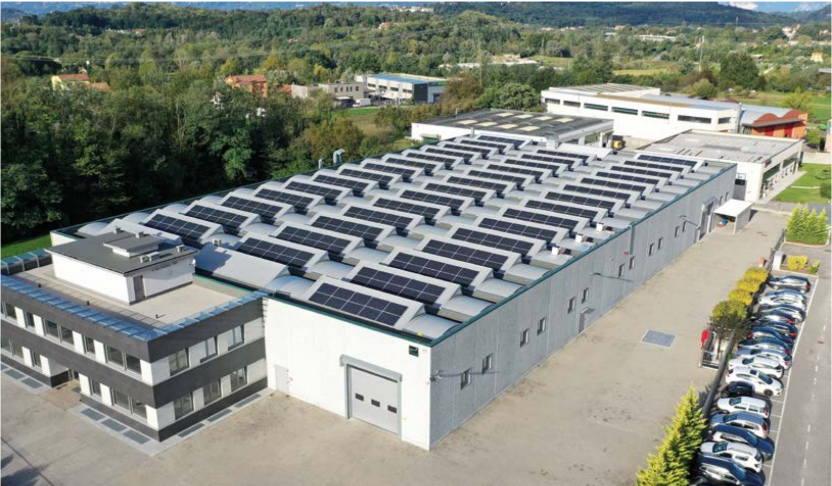
.6 Stabilimento di Cocquio Trevisago | Cocquio Trevisago Production Plant
